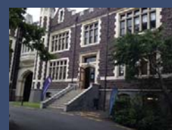
International Division Archway West building
