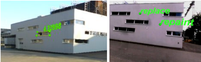
Fig. 22. Interactive techniques. Left) AR surveying of a window. Right) AR annotations used to store annotations spatially aligned to the building.
