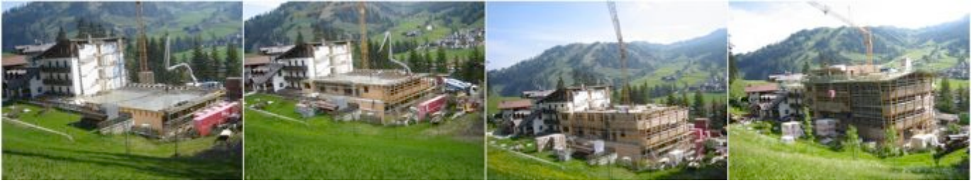
Fig. 1. Construction site monitoring using camera images. The image sequence represents different steps of the construction progress. This information can be difficult to analyze and search for sources of mistakes. Furthermore, it is tedious for the user to map the 2D camera image information into the actual physical 3D environment.
